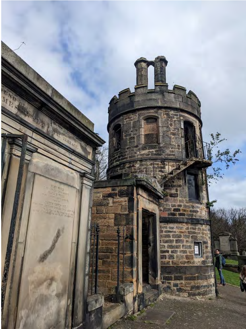
Watch Tower from west
